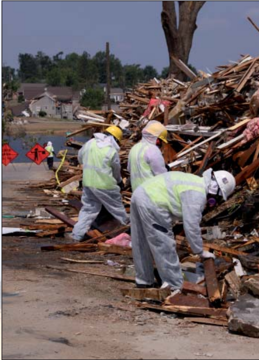
A segregation crew separating debris that contains asbestos.
