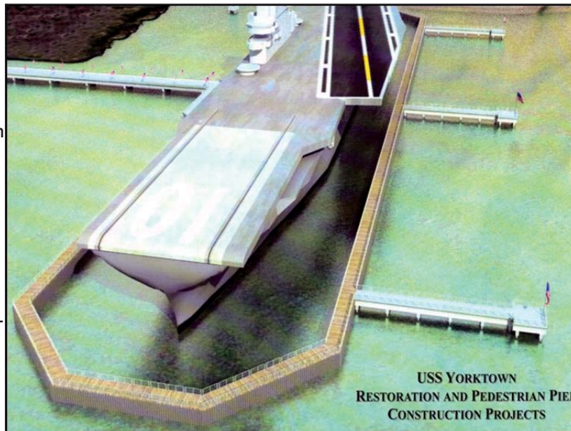
This rendering shows how a permanent cofferdam would look around the USS Yorktown .
