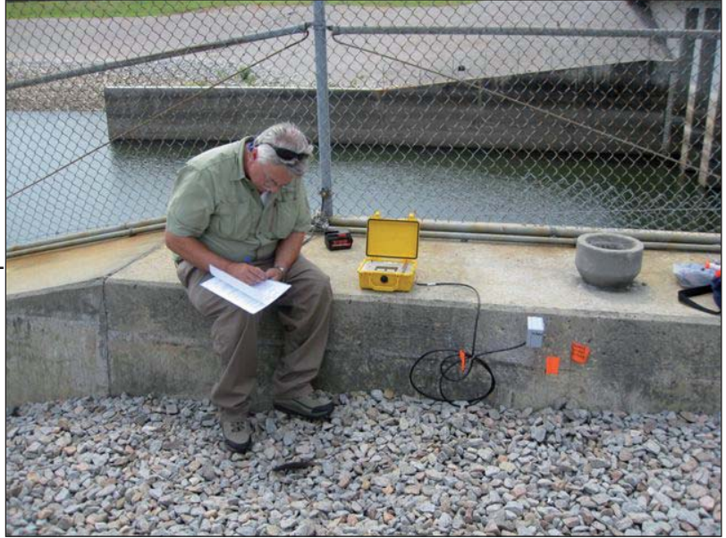
Tommy Socha installs a tilt meter monitoring system at the powerhouse. The tilt meter will electronically monitor movements in the spillway during facility operations during the year and is another way the District works to keep safety the number one priority in all activities.
